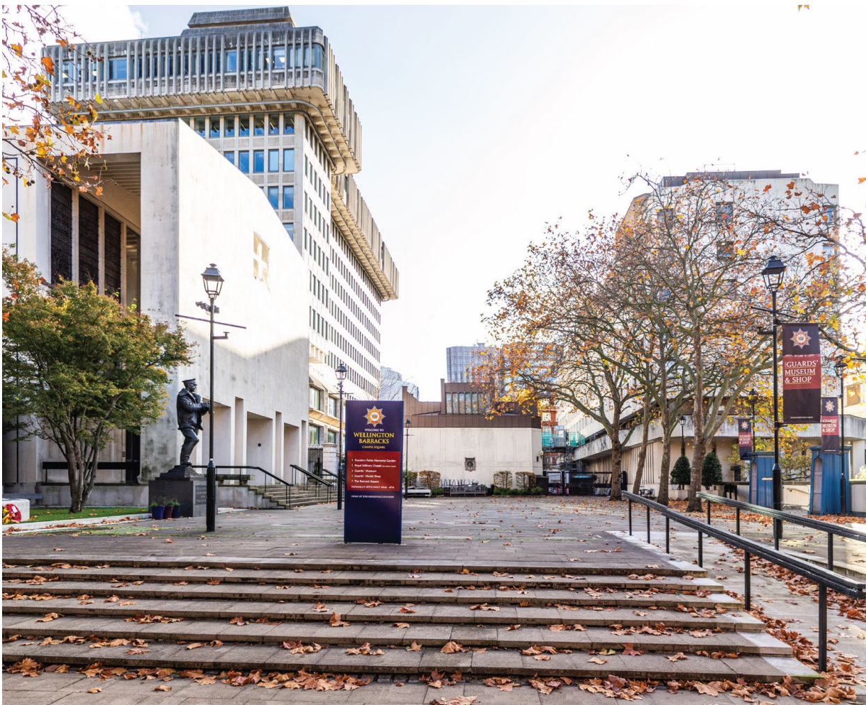
View from within Wellington Barracks towards the Rehearsal Hall, Barracks Accommodation, and adjacent Ministry of Justice
